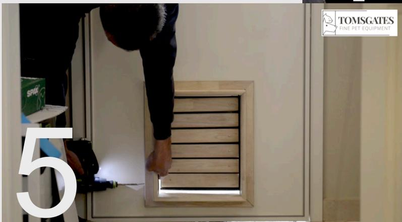
**slide up and tighten the inner frame**
